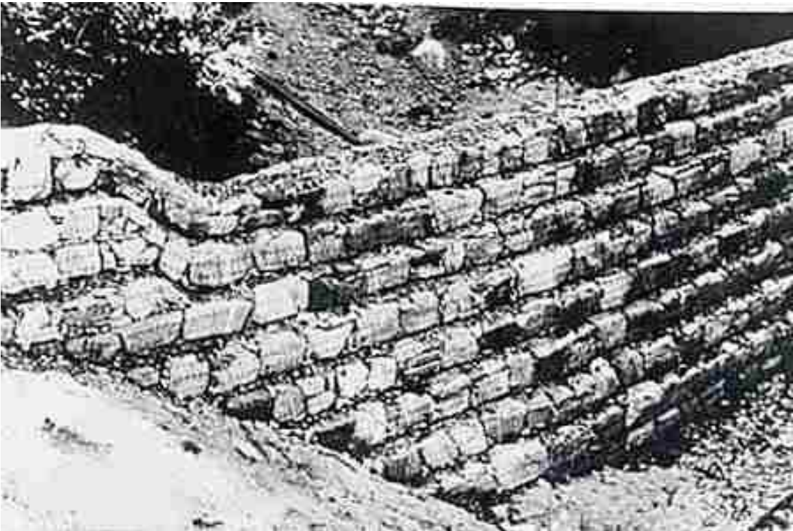
Figure 5.37. Gabion debris dam.
