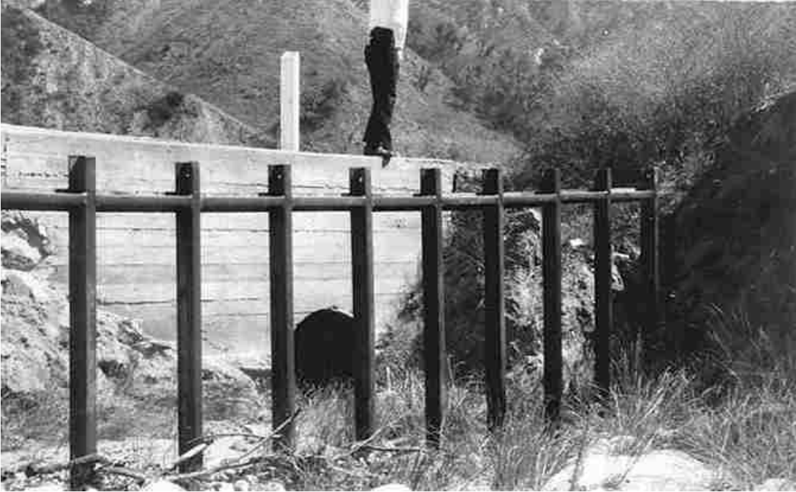
Figure 5.12. Rail debris rack.
