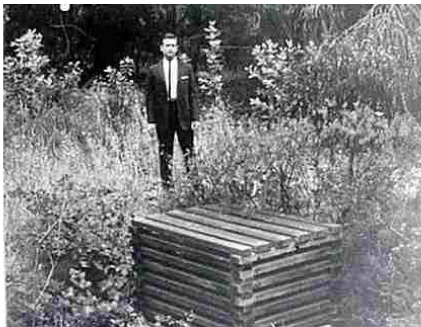
Figure 5.28. Redwood debris crib with spacing to prevent passage of fine material. Basin had buildup of 30 feet.
