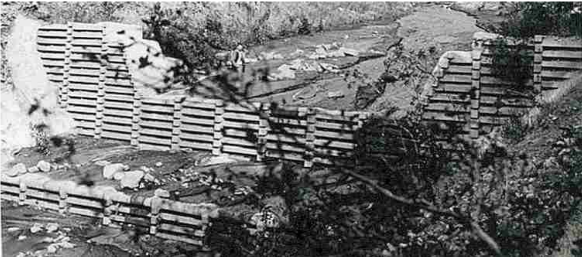
Figure 5.38. Debris dam of precast concrete sections fabricated to enable placement in interlocking fashion.
