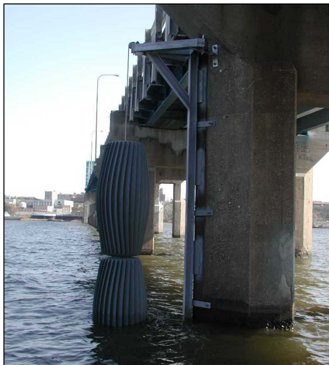
Figure 5.47. Close up of double-stacked installation debris sweeper on Interstate 24 over the Mississippi River.
