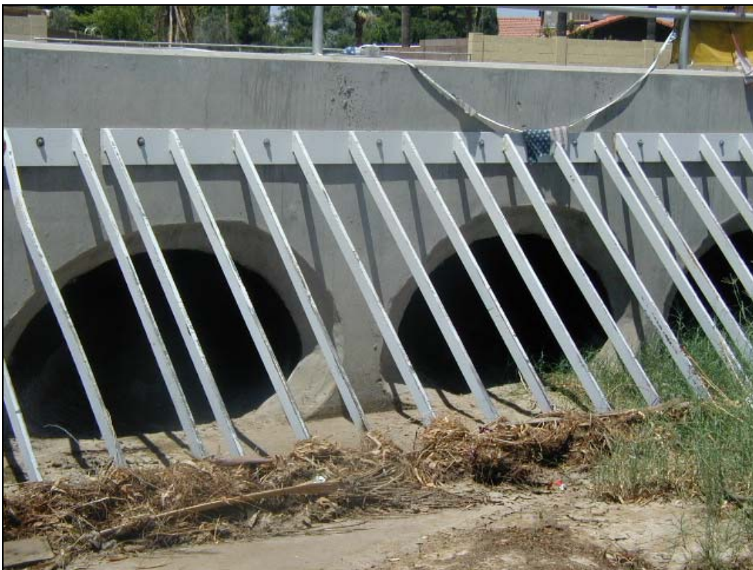
Figure 5.15. Steel debris rack in urban area.
