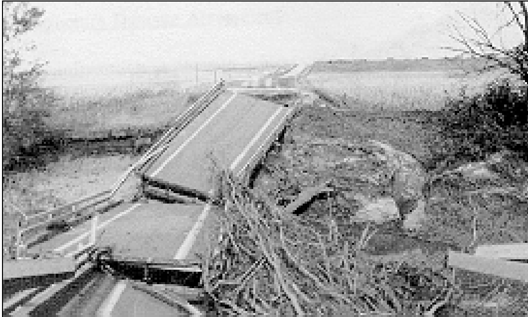
Figure 2.4. Missouri Highway 113 bridge over Florida Creek near Skidmore, Missouri.
