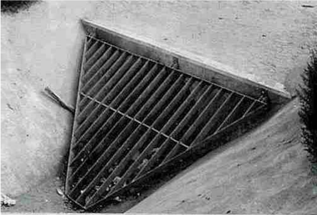
Figure 5.14. Hinged steel debris rack in urban area. Due to nature of debris and possible entry by children, bar spacing is close.
