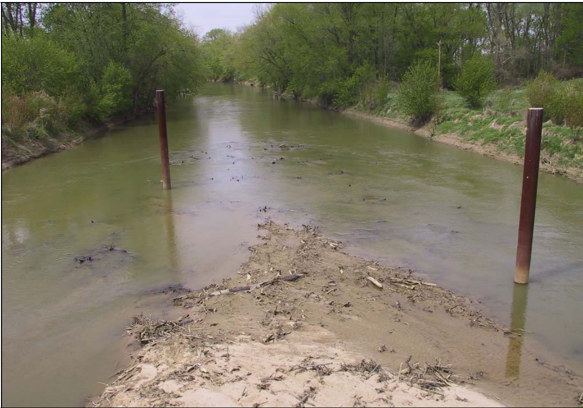
Figure 5.43. Debris deflectors installed at State Route 59 south crossing of the Eel River in central Indiana.
