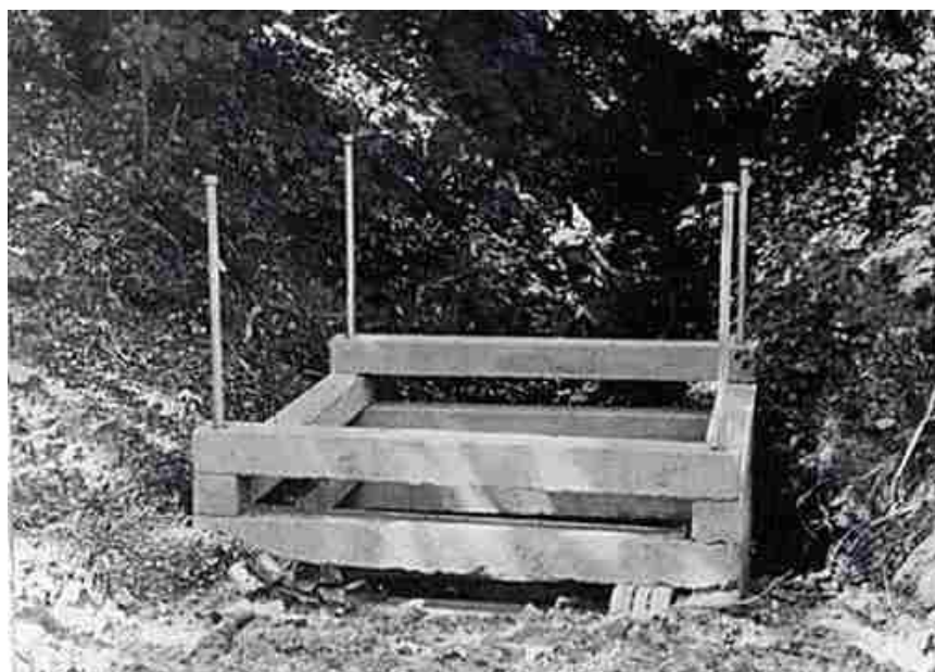
Figure 5.26. Debris crib of precast concrete sections and metal dowels. Height increased by extending dowels and adding more sections.
