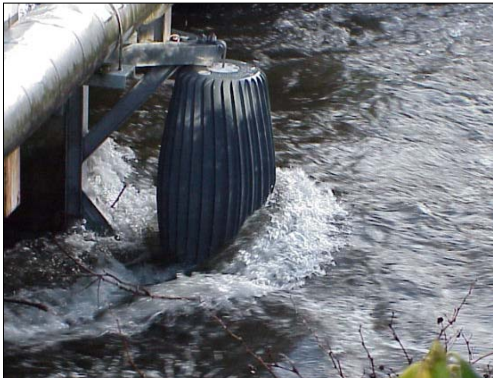
Figure 5.45. Close up of a debris sweeper installed on the Cedar Creek in Washington.
