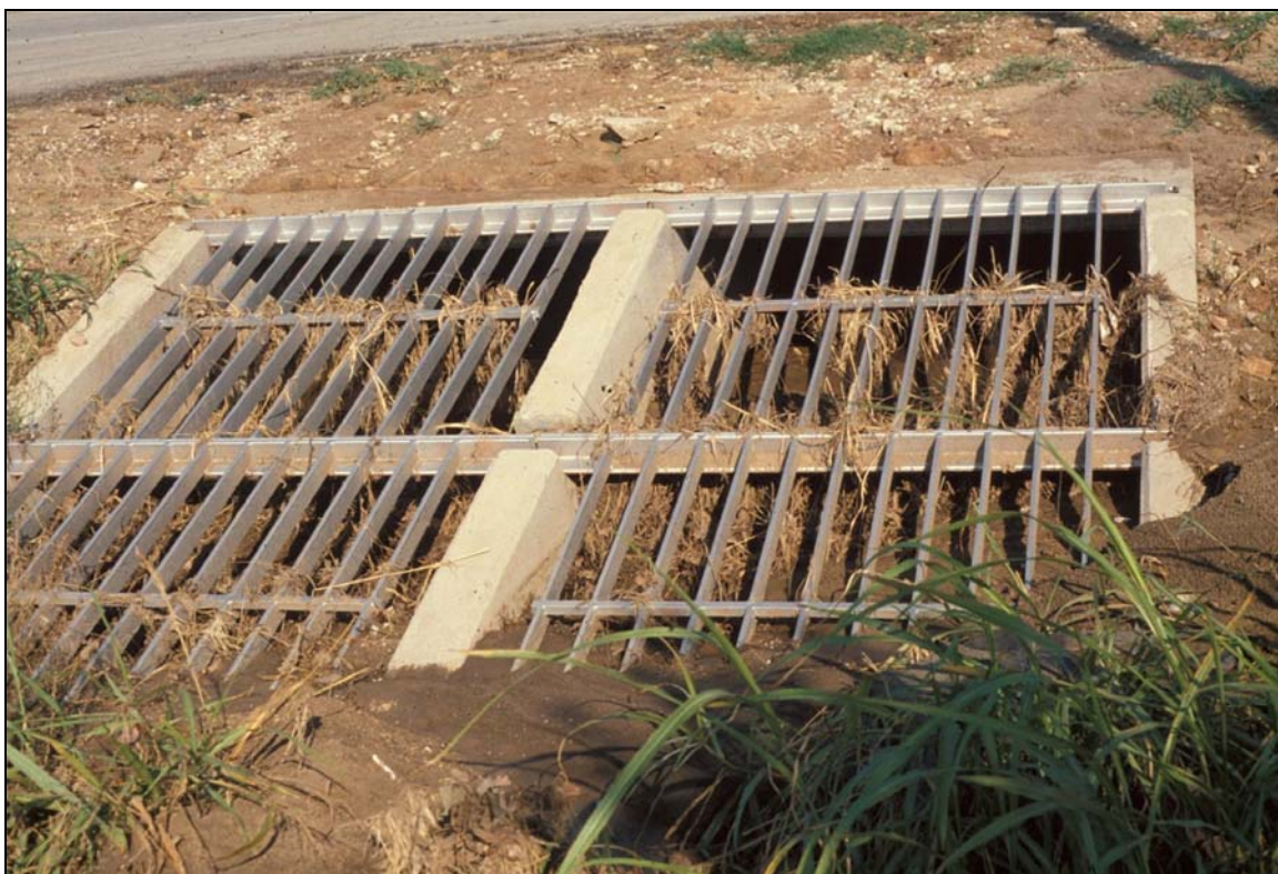
Figure 5.22. Steel grill debris rack on slope mitered culvert entrance.
